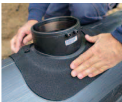
The self-adhesive rubber mat seals the saddle on an ASA VL d160 pipe.
