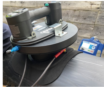
The vacuum is maintained while fusing.
